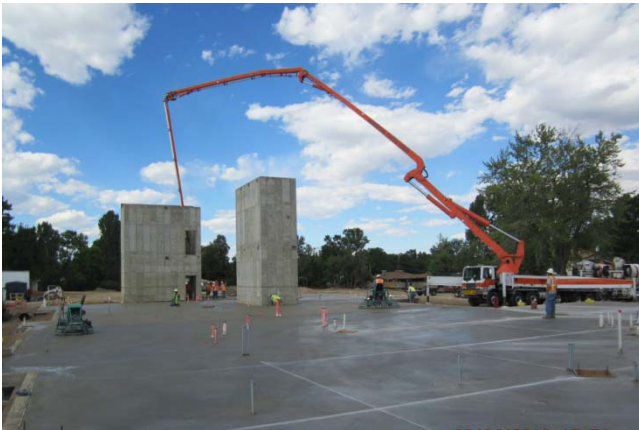
Construction proceeds on JFHSC site
