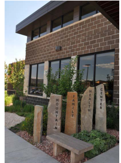
The new Mountain Family Health Center in Rifle.
