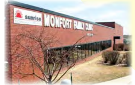
Sunrise Community Health, Inc., which cared for more than 22,000 people in 2007, opened its new Monfort Family Clinic in Evans in July 2007. The new building replaced a 1915 schoolhouse-turned-Community-Health-Center in Greeley. Community donors and foundations provided the capital investment, knowing that Sunrise's PCF dollars would help to staff and operate the new facility.
